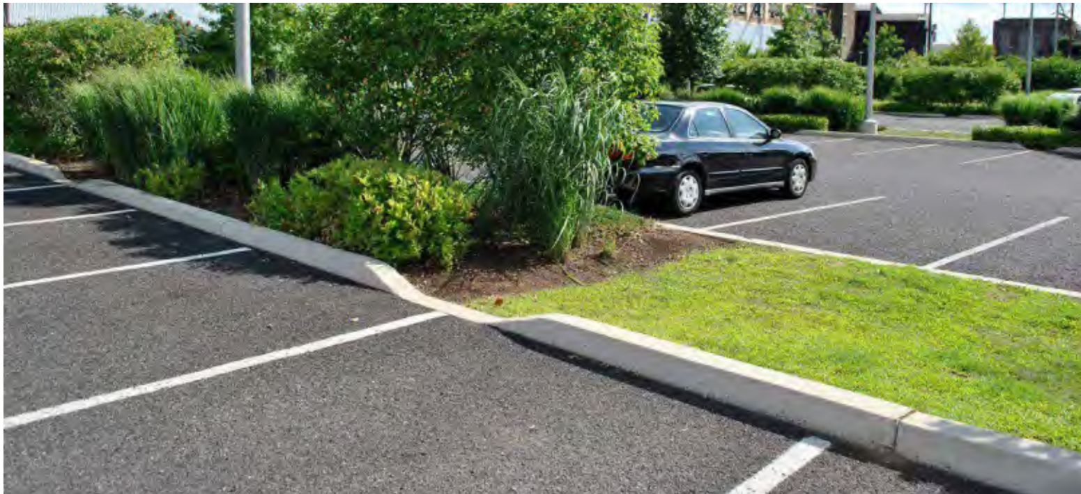
A bioretention practice in Philadelphia, PA, with a wide curb opening and angled edges to facilitate runoff capture.
