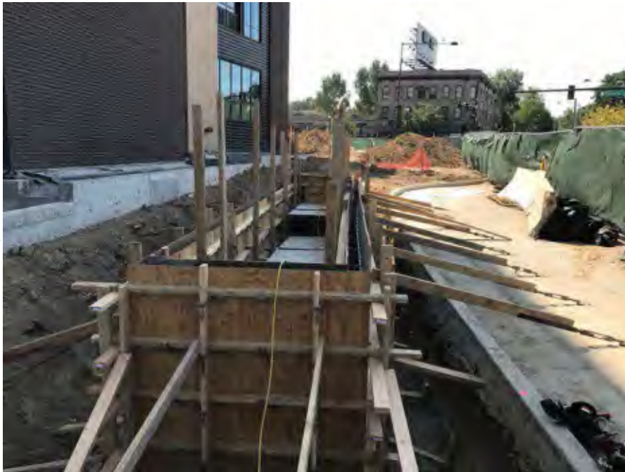
Bioretention under construction in Denver, CO.
