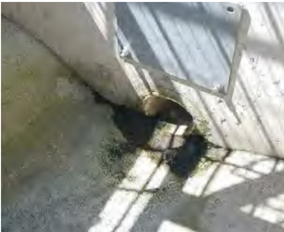
Underdrain outlet in an outlet box.
