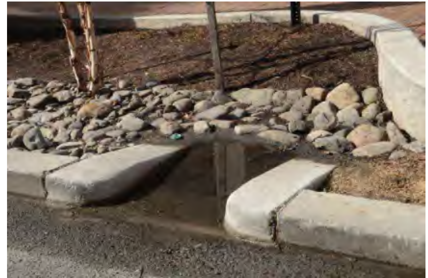
Incorrectly installed inlet.
