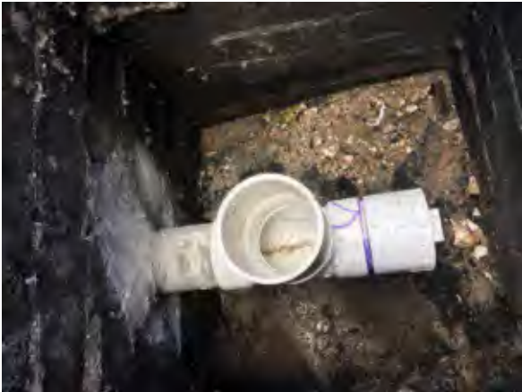
An IWS system with an outlet box.
