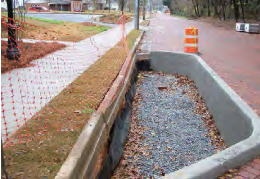
Bioretention under construction in Atlanta, GA.
