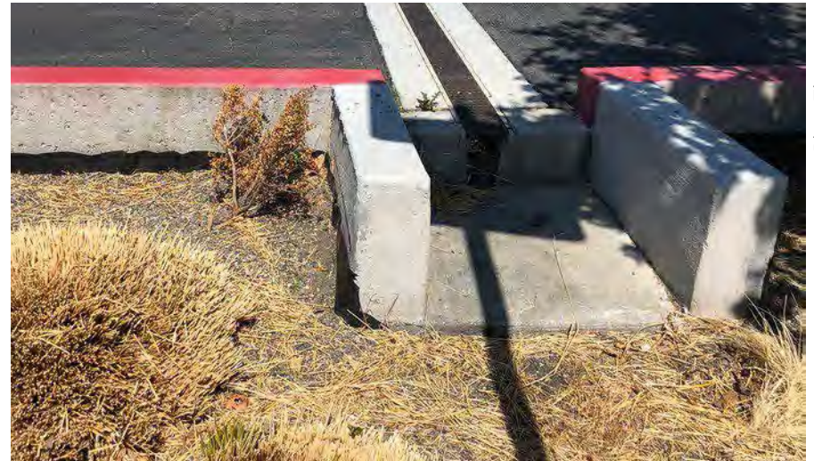
Concrete splash pad in San Mateo, CA
