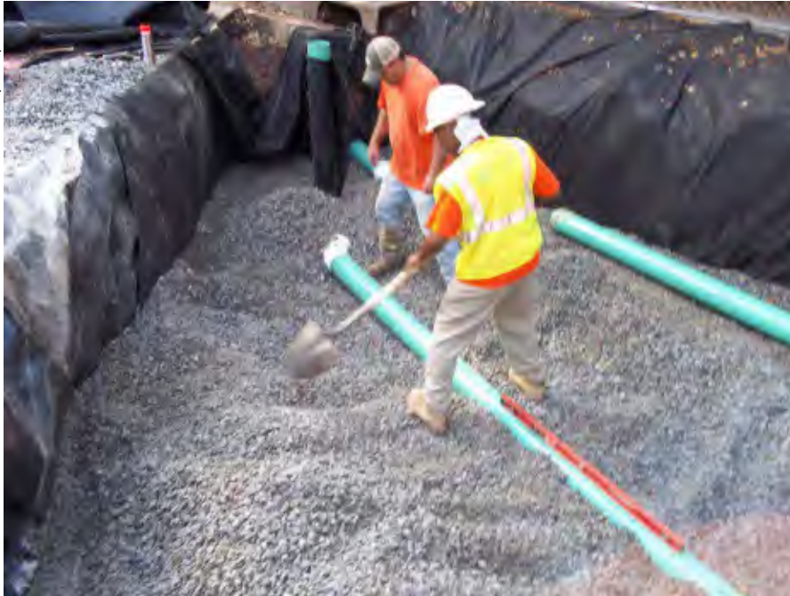
Installing aggregate media in Atlanta, GA.
