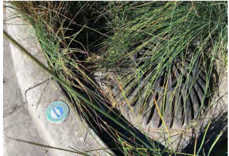
Vegetation overgrowth is blocking an overflow structure.
