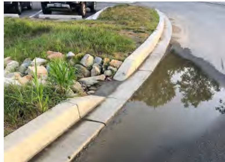
Improper grading causes water to build up at the edge and not flow into this facility.
