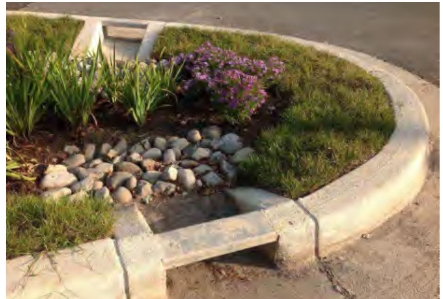
Wheel guards protect openings from vehicles on this stormwater curb extension in Montgomery County, MD.
