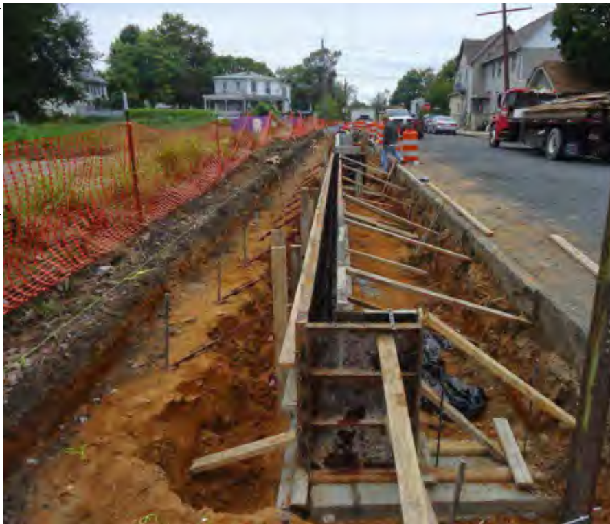
Bioretention under construction in Camden, NJ.
