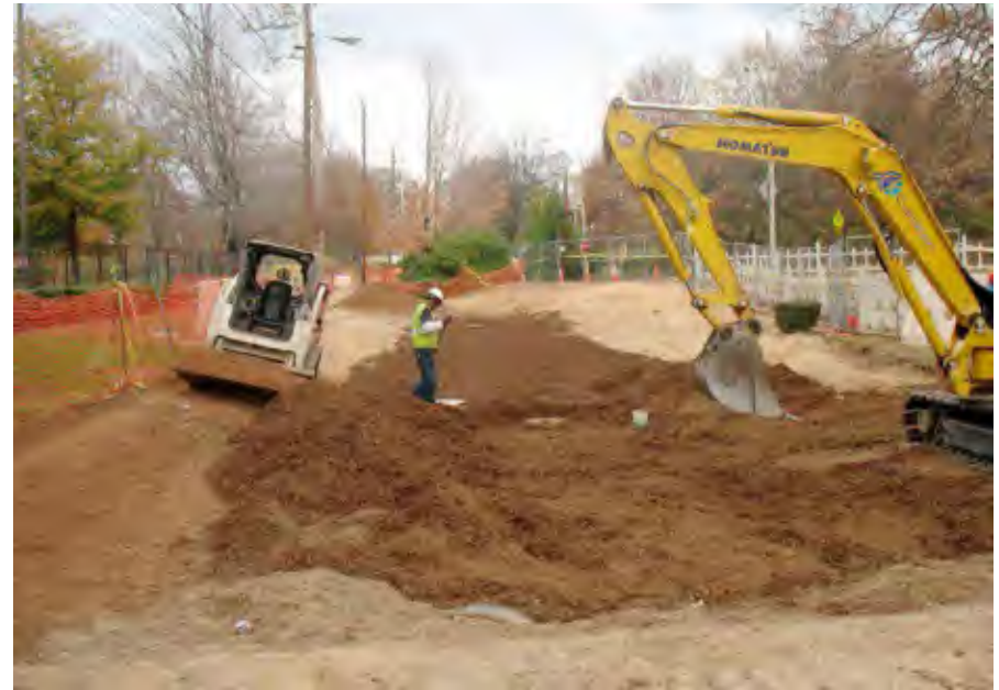
Bioretention facility under construction in Atlanta, GA.
