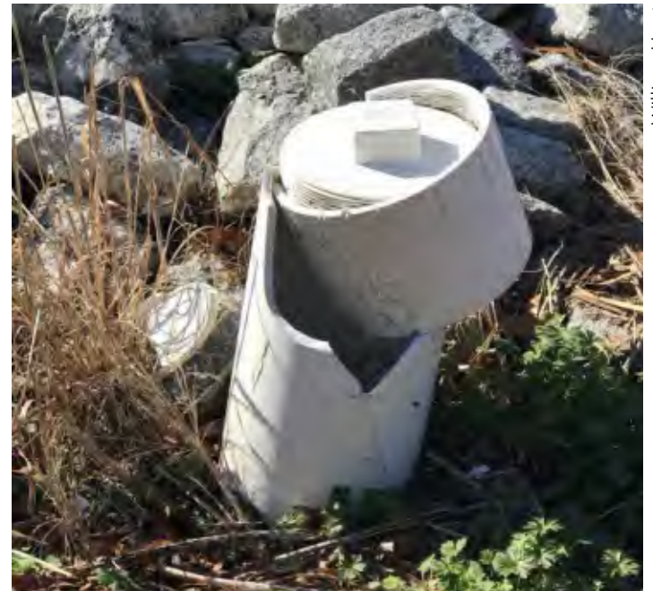
A broken cleanout.
