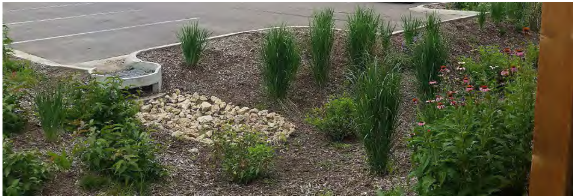
Inlet sump forebay paired with a rock forebay in Minneapolis, MN.
