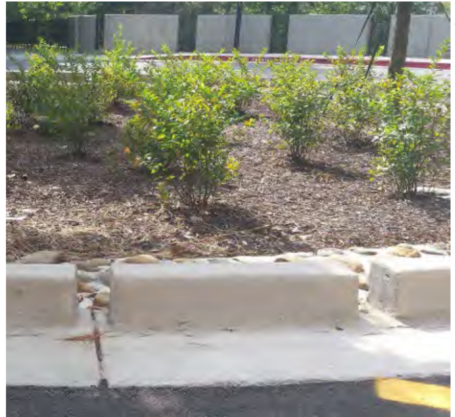
Small inlet openings convey runoff into a bioretention practice within a traffic median in Atlanta, GA.
