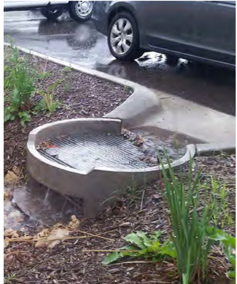
Proprietary inlet sump in Minneapolis, MN.
