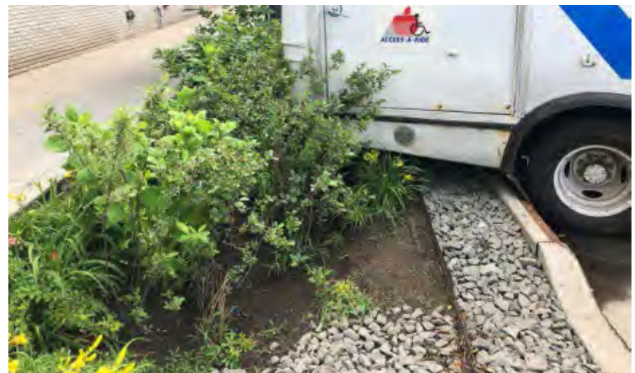
A vehicle backed into a bioretention practice lacking adequate protection.
