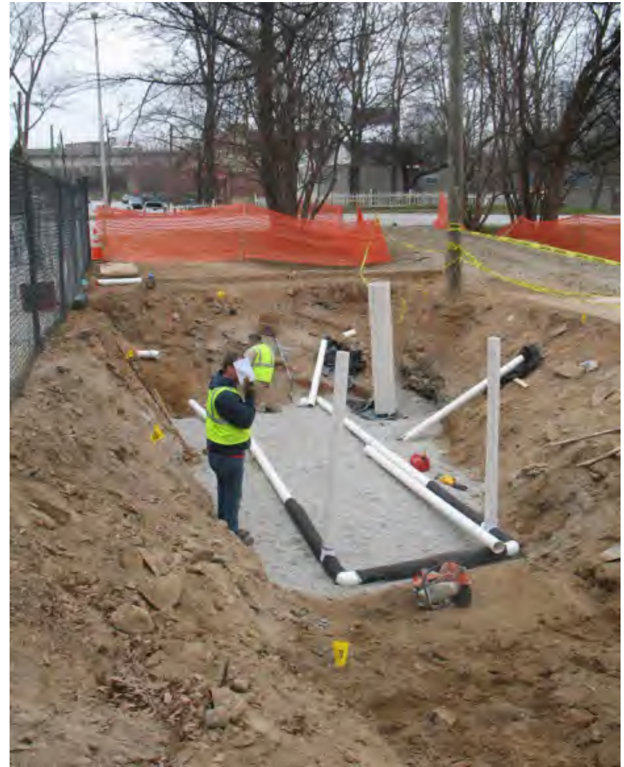
Bioretention under construction in Atlanta, GA.
