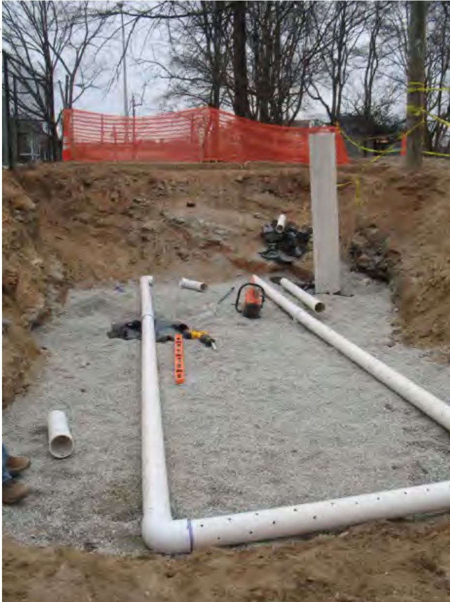
Underdrains being installed in Atlanta, GA.
