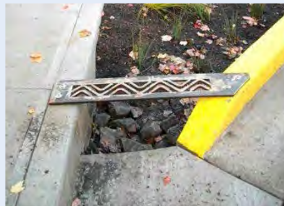
Metal bars added across inlet opening prevents vehicle access.
