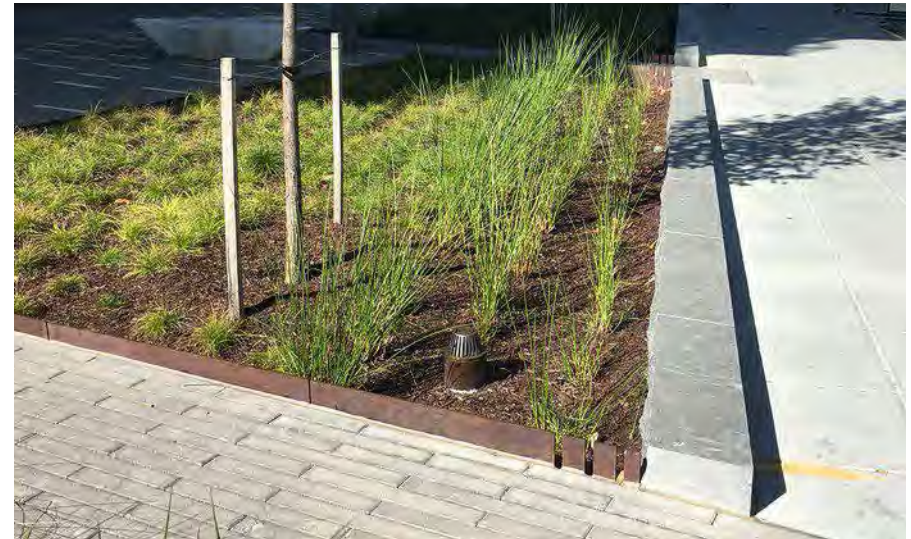
A highly visible bioretention area that has clearly marked plant groupings for easy maintenance in Washington, DC.
