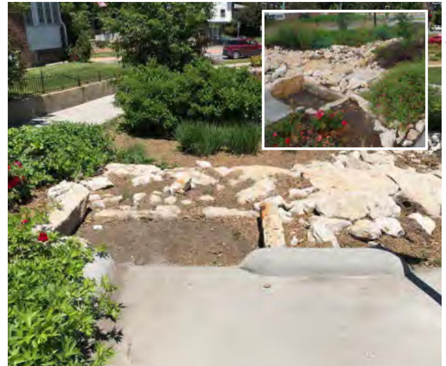
A limestone forebay captured significant amounts of sediment (see inset for typical depth of a newly installed forebay) and needs maintenance in Omaha, NE.
