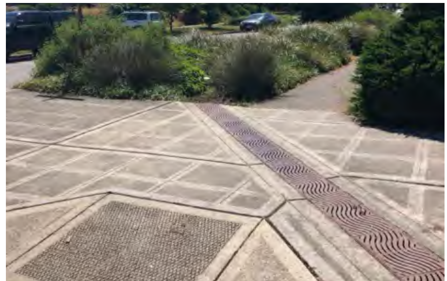
A trench drain allows for runoff conveyance and pedestrian circulation in Seattle, WA.
