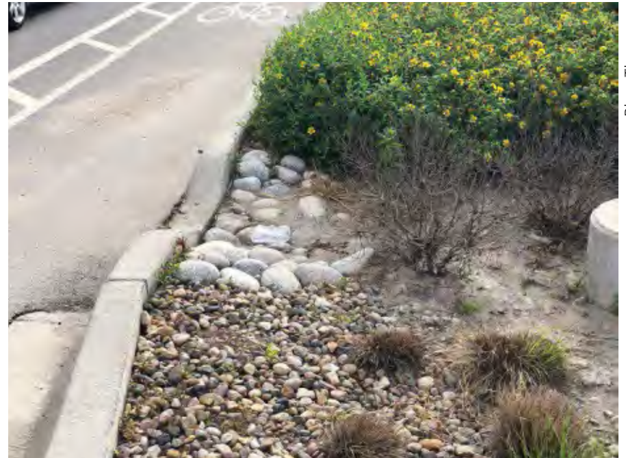
A sediment-clogged stone forebay.
